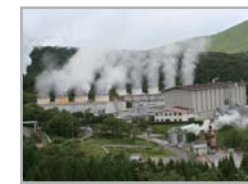
Hachobaru Power Plant (Learn about Geothermal Energy)
